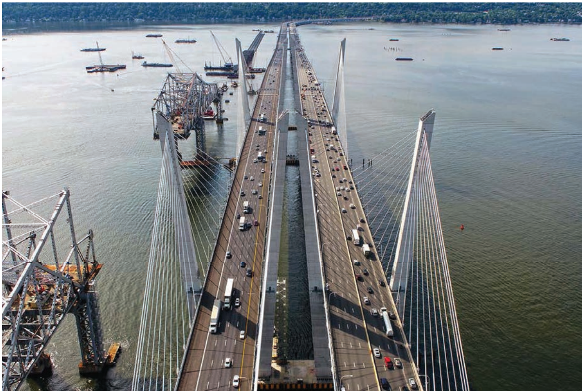
Figure 12: New NY Bridge Project
